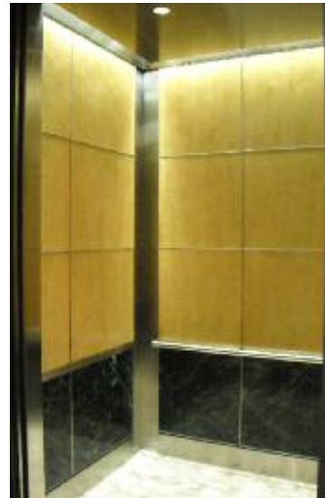
1515 Wynkoop: lower panels in Verde Antique stone; upper panels in Curly Maple wood veneer; inlay in Satin SS; Custom Satin SS ceiling with LED perimeter lighting; custom handrail
