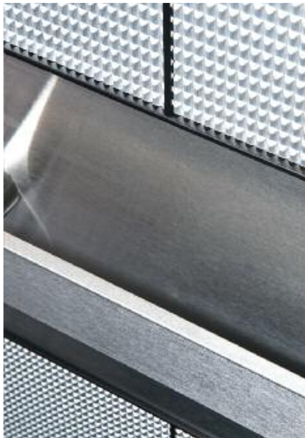
Sahara I: layer 2 & 4 in Museum (Nickel); layer 3 in Satin SS; Aluminum Inlay in Black Anodized Aluminum; 2" flat handrail
